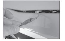
**132.** Mix 1/2 ounce (15ml) of 30-minute epoxy. Use an epoxy brush to apply epoxy in the tubes in the fuselage for the fin and to the surrounding wood.
